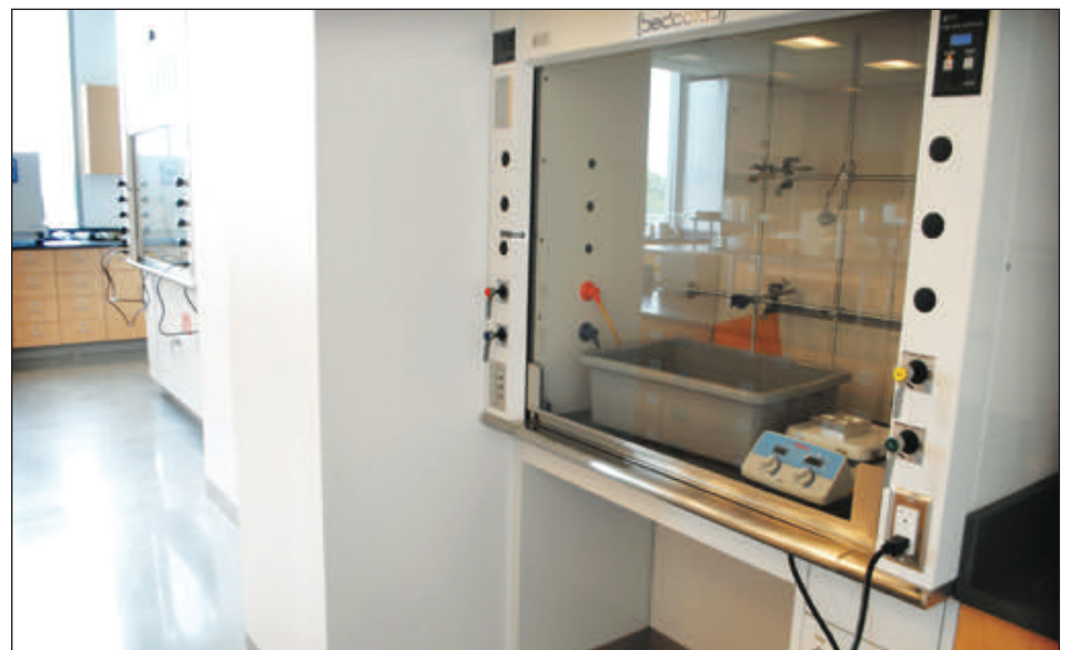
Laboratories in the Keck Center have wheelchair-accessible fume hoods and other disability-friendly features.
